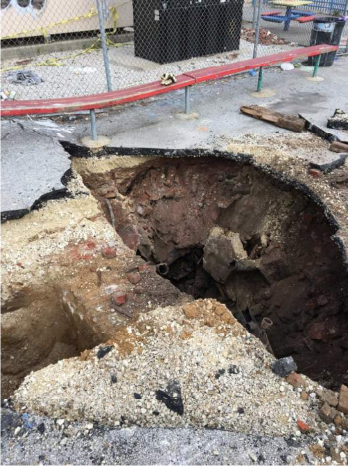
Test Pit #1, April 19, 2017
