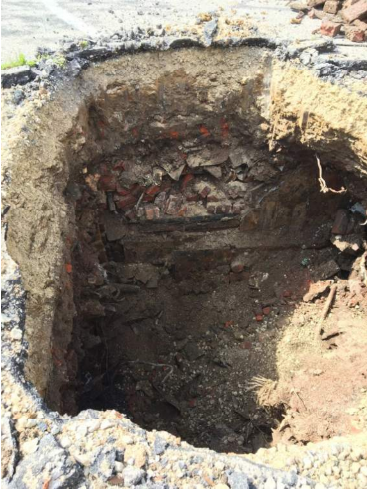
Test Pit #2, April 19, 2017
