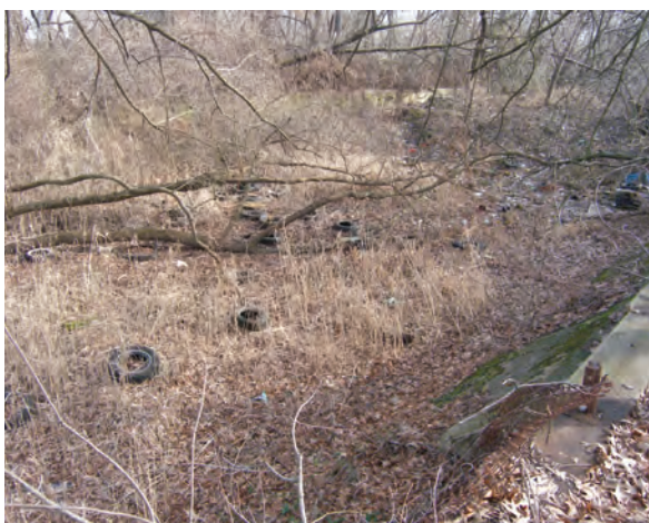
Above: Images of abandoned channel infrastructure near 84th and Mario Lanza Boulevard, 2013
