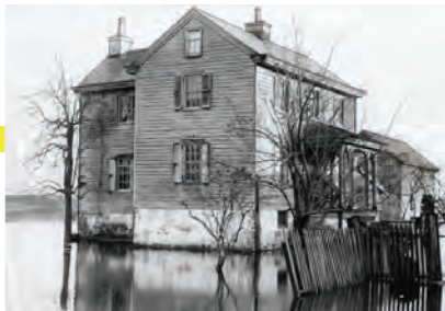
Eastwick section partly inundated by bow creek
